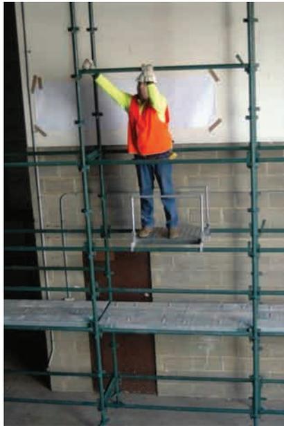
**Figure 5: Photographic illustration of erection and dismantling using two erection platform options for a three plank wide scaffold. Note: scaffold is shown against a building, so guardrails only needed on external face. Toeboards and lower mid-rails omitted for clarity.**
