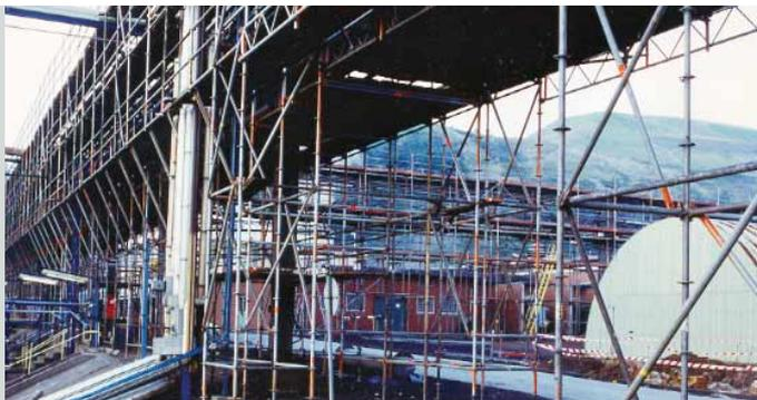
The Layher Allround System in steel with its highly functional components permits complex and very difficult scaffolding structures to be built.
