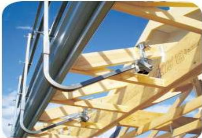
TYPE 1: L BEND EXPOSED EAVES
